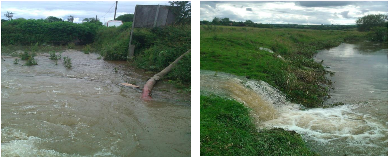
Figure 24 – Derwent North main failure at River Teams, 2010.
