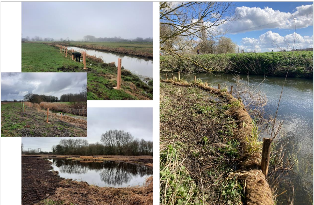
Tree planting, wetland scrape creation and installation of coir matting along the riverbank
