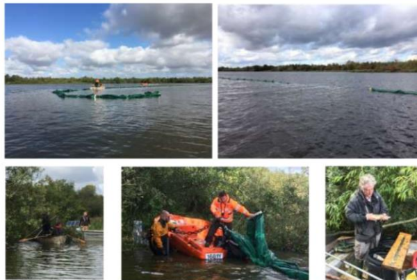
Ranworth broad fish barrier installation and biomanipulation
