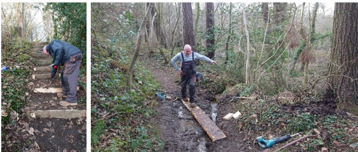
Step and drainage improvements at Ulgham LNR
