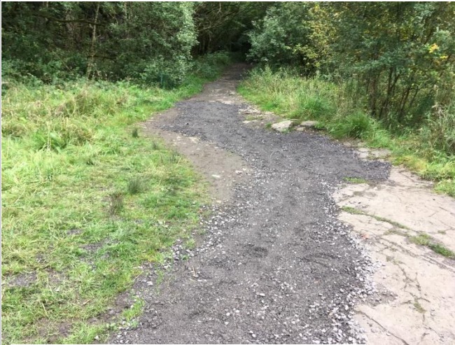
Some fresh resurfacing on Trammer Trail 3
