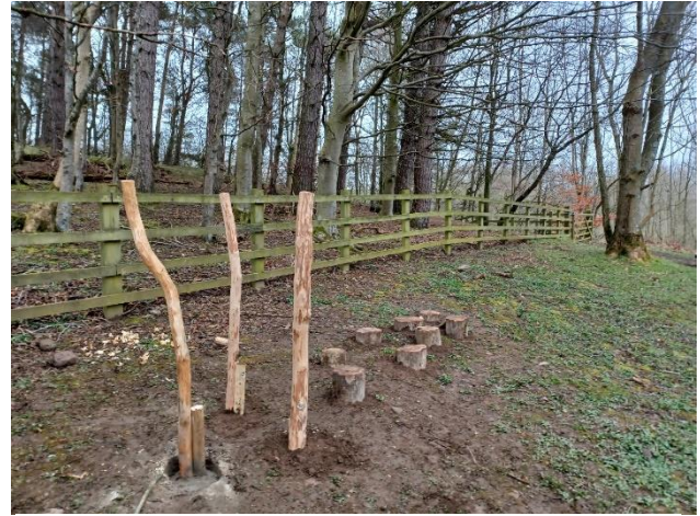
The play area during construction
