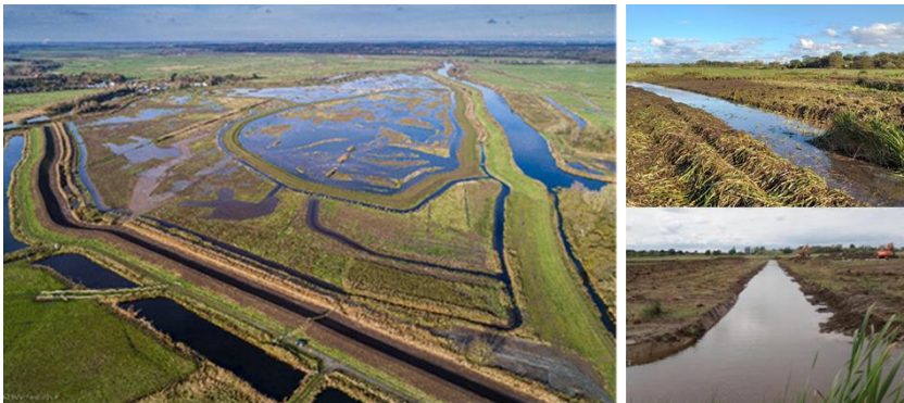
Extensive areas of wetland scrapes, pools, dykes and marsh created at Carlton Marshes
