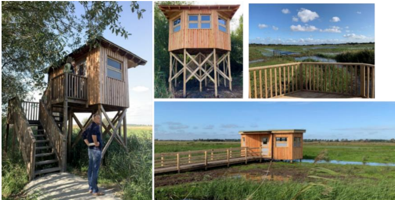
Carlton Marshes viewing hides and structures
