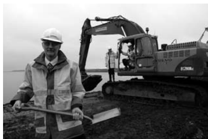
Work begins at Abberton Reservoir
