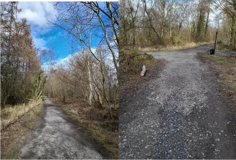
Path resurfacing works
