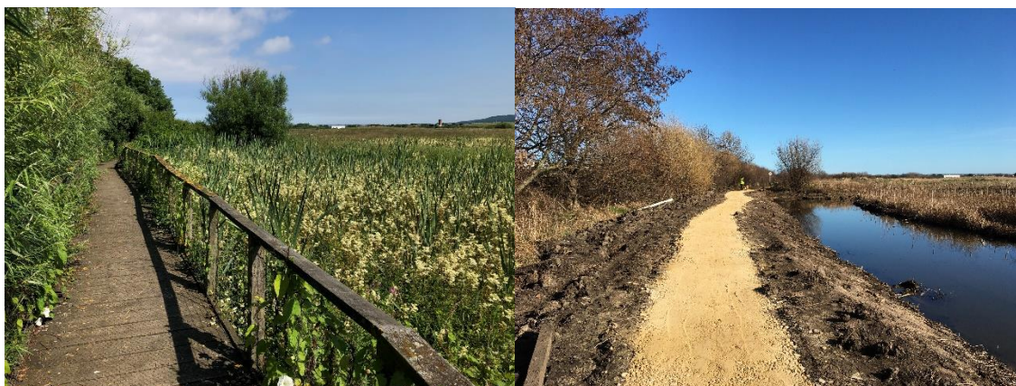
Coatham Boardwalk before and after removal, earthworks, and resurfacing
